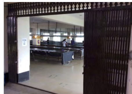
Before remediation (left) – collapsible gate; After remediation (right) – fire door installed
