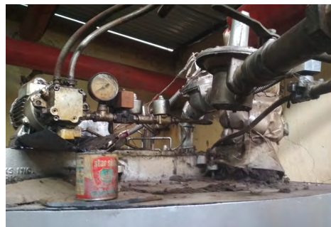
Left: Inadequate remediation of leakage from boiler shell by using clay; Right: Leakage on input fuel line - constitutes risk of explosion
