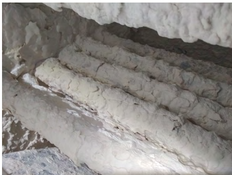
Corrosion of the boiler wall due to calcium build-up; this can reduce the efficiency of the boiler and lead to leakage of boiling water.
