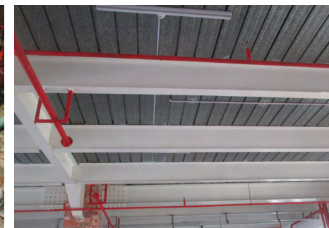
Installation of fire protection systems: hydrant system (left) and sprinkler system (right)
