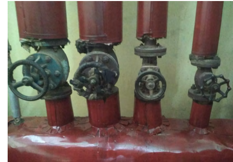
Left: Uninsulated steam valves and flanges - increases the scorching risk for operators; Right: Rusty weld joint & symptoms of unburnt fuel - reduces efficiency and causes risk of explosion
