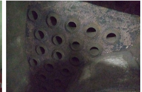
Left: Uninsulated steam valves and flanges - increases the scorching risk for operators; Right: Rusty weld joint & symptoms of unburnt fuel - reduces efficiency and causes risk of explosion
