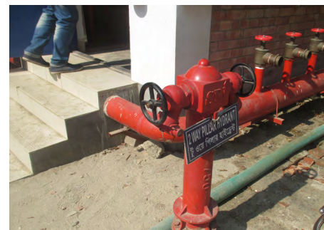
Installation of fire protection systems: hydrant system (left) and sprinkler system (right)
