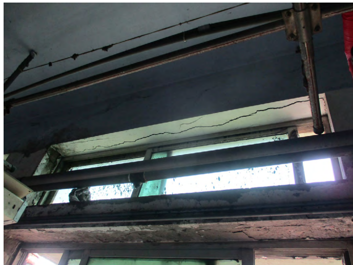
Findings: excessive wall cracks and cracks in beams and ceiling slabs
