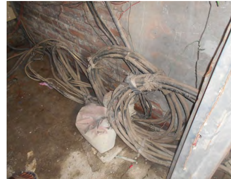
Before remediation (left) – unsupported and unsafe cables; After remediation (right) – cables are adequately supported; cable tray installed
