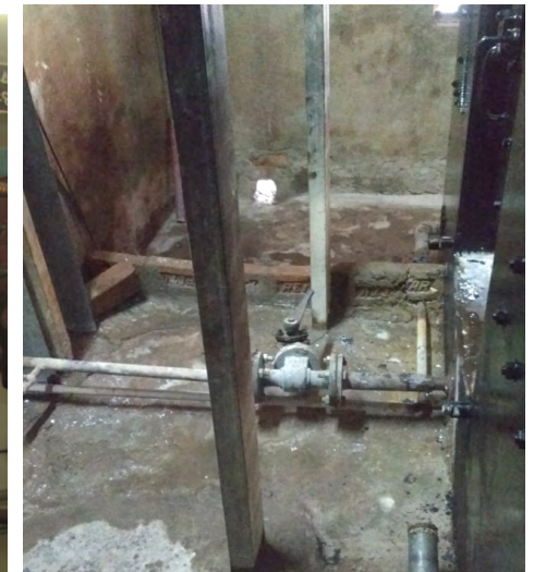
Left: Faulty electrical wiring - makes the boiler unsafe to operate & constitutes a fire hazard; Right: Rusty blow down pipe - can cause leakage, increasing the scorching risk for operators
