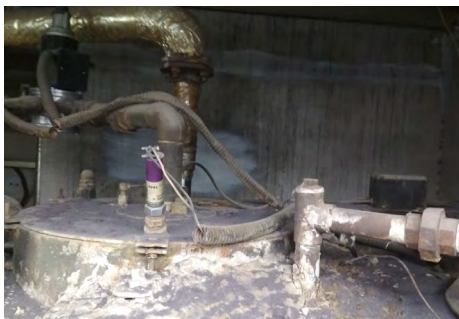
Left: Inadequate remediation of leakage from boiler shell by using clay; Right: Leakage on input fuel line - constitutes risk of explosion
