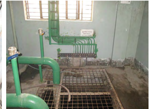
Before remediation (left) – unsupported and unsafe cables; After remediation (right) – cables are adequately supported; cable tray installed
