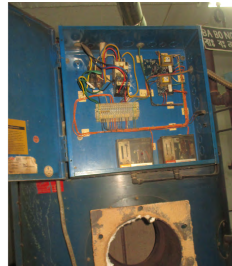
Left: Faulty electrical wiring - makes the boiler unsafe to operate & constitutes a fire hazard; Right: Rusty blow down pipe - can cause leakage, increasing the scorching risk for operators
