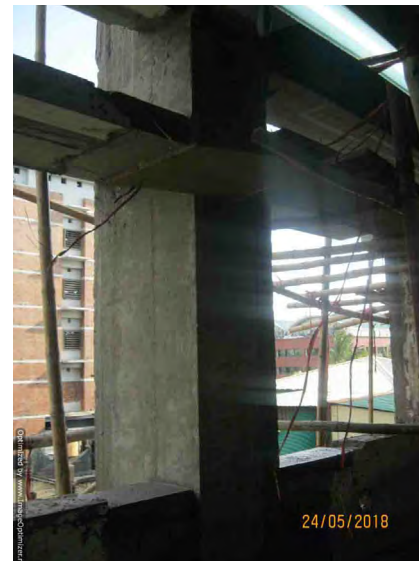
Structural retrofitting ongoing. After the structural remediation had been verified as completed, the factory was determined safe for re-occupation and resumption of production.
