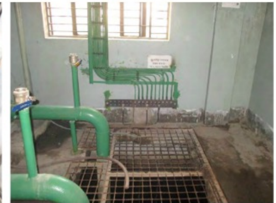
Before (left) – unsupported and unsafe cables; After (right) cables with adequate support, cable tray installed
