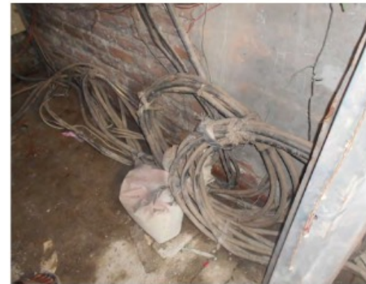
Before (left) – unsupported and unsafe cables; After (right) cables with adequate support, cable tray installed
