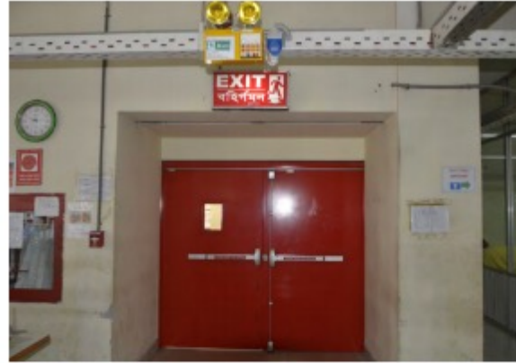
Before (left) – collapsible gate; After (right) fire door installed
