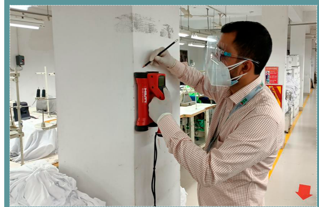
An RSC engineer performing a structural safety inspection using a ferro scanner to assess the strength of a factory building's column. Photo credit: RMG Sustainability Council (RSC).
